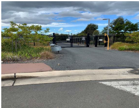
Image 1: Access to Leppington Stabling Yard off McCann Rd
