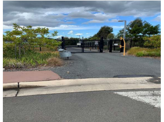
Image 10: Access gate N06 53.257 D to rail corridor via Leppington Stabling Yard carpark
