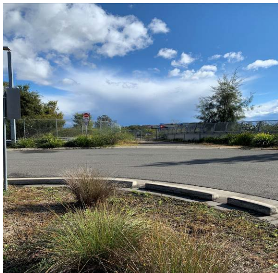
Image 5: Access Gate into rail corridor from Leppington Carpark
