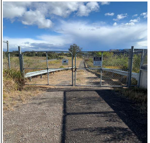
Image 6: Access Gate into rail corridor from Leppington Carpark
