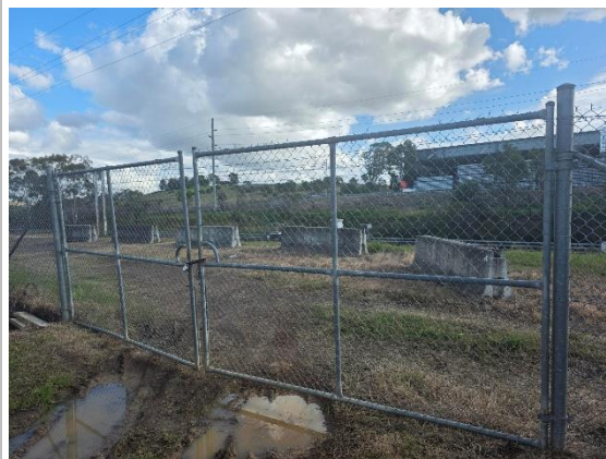
Image 3: Access gate NO: SOO 47.629 D countryside of Ingleburn Station.
