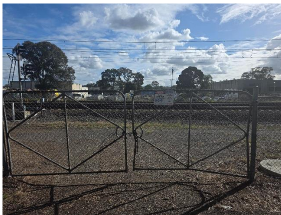
Image 1: Access gate NO: SOO 46.304 D countryside of Ingleburn Station.
