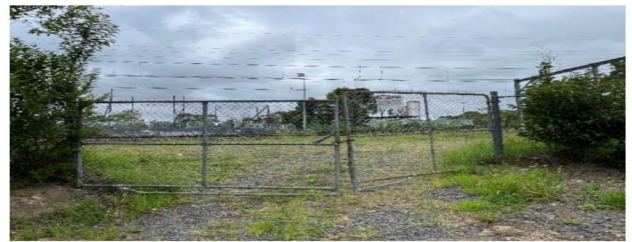
Image 2: Sensor access using access gate N00 30.700 D
