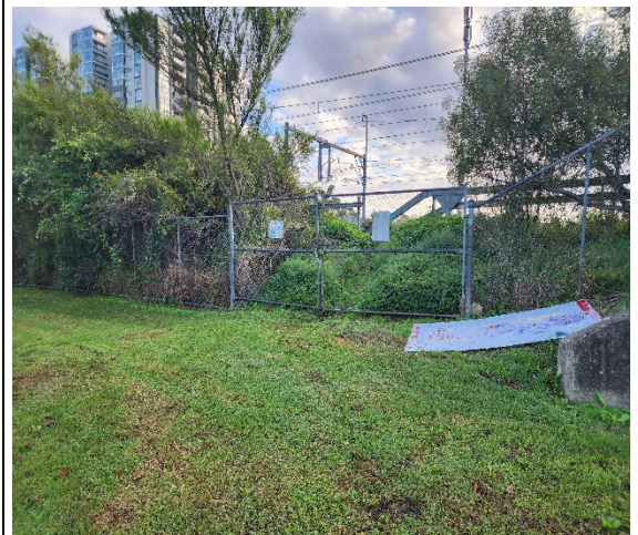
Image 6: Access/Egress gate M00 20.922D on Memorial Drive, City side of Granville station
