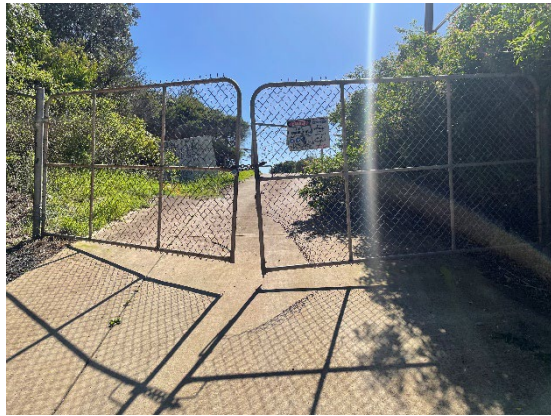
Image 1: Access gate 100 58.463 Worksite and Coalcliff Side Protection Access and Egress (Lawrence Hargrave Dr)
