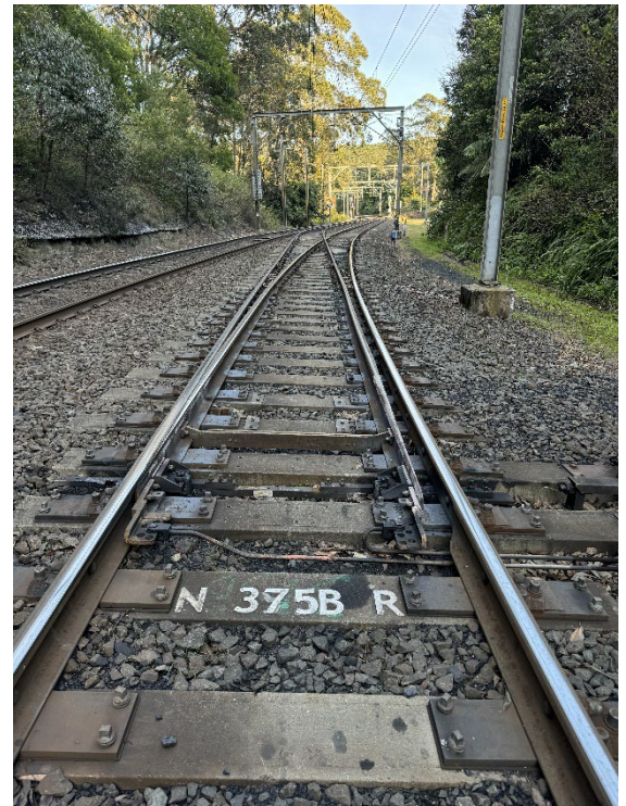
Image 7: 375 B Points – Clip and Lock Normal
