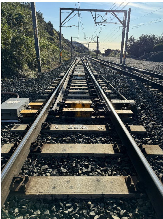
Image 8: 367 A Points – Clip and Lock Normal
