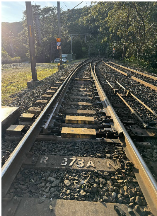
Image 6: 373 A Points – Clip and Lock Normal
