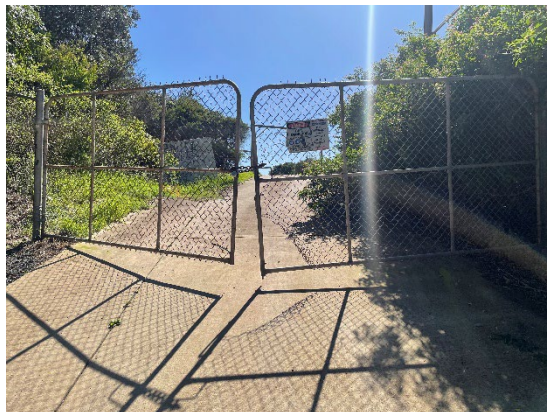
Image 1: Access gate I00 58.463 Worksite & Coalcliff Side Protection Access and Egress (Lawrence Hargrave Dr)
