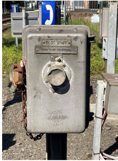
Image 3: Half Pilot Staff Coalcliff to Otford Up WG 660 U Worksite end of Coalcliff Platforms
