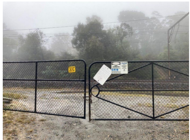
Image 2: Sensor access using access gate W00 101.891 U
