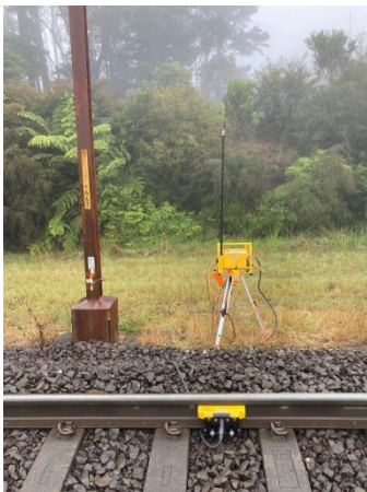
Image 1: Sensor and transmitter installation location
