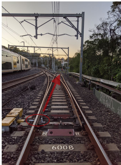
Image 3: 600 points clipped and locked to prevent rail traffic entering the worksite
