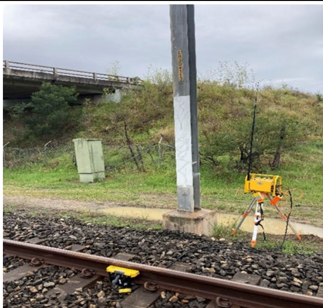
Image 1: Transmitter and sensor installation location
