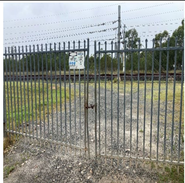
Image 2: Sensor access gate M25 30.049 U
