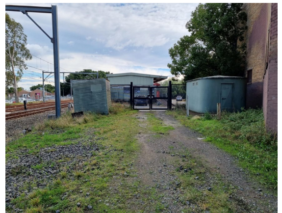
Image 6: Access gate M24 18.965 to access 361 points and 362 points .
