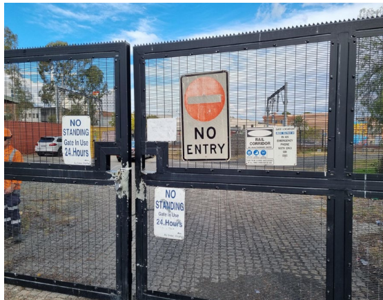
Image 5: Access gate M24 18.965 U – Depot PI via Marion St.
