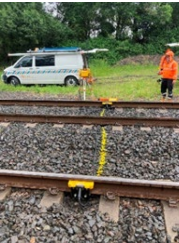
Image 1: Transmitter and sensor installation location
