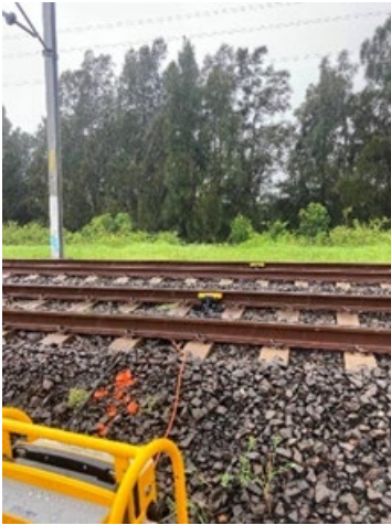
Image 1: Transmitter and sensor installation location
