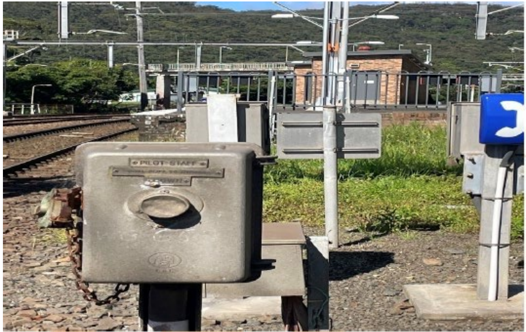
Image 4: Half Pilot Staff Coalcliff to Otford Down (Off the Otford end of Coalcliff Platform)
