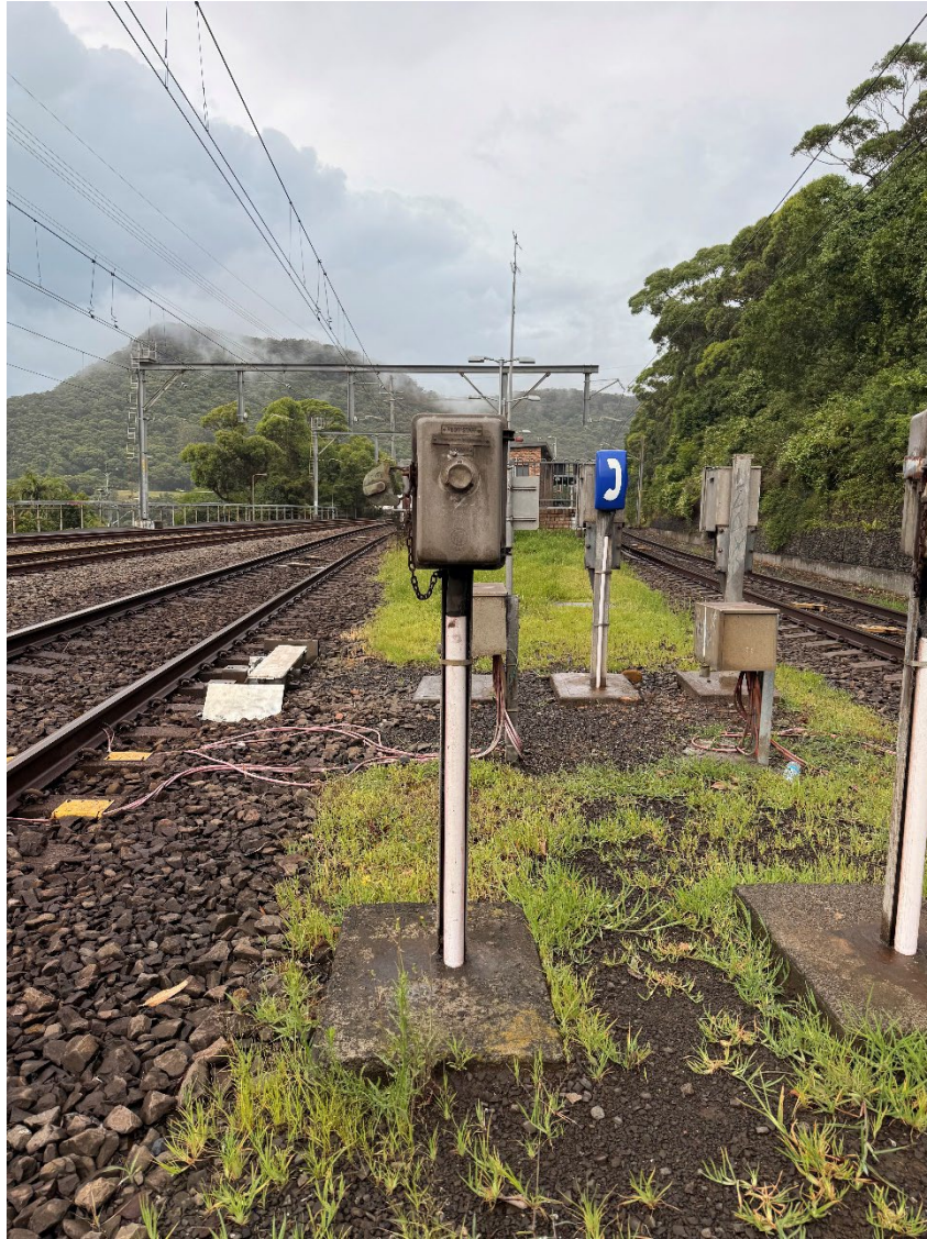
Image 1: Half Pilot Staff Coalcliff to Otford Down (Off the Otford end of Coalcliff Platform)
