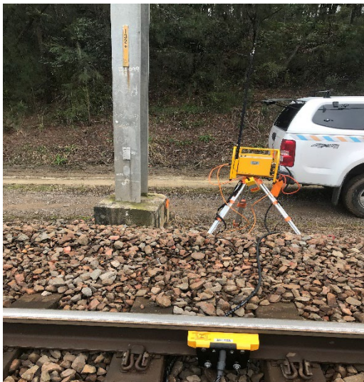
Image 1: Transmitter and sensor installation location
