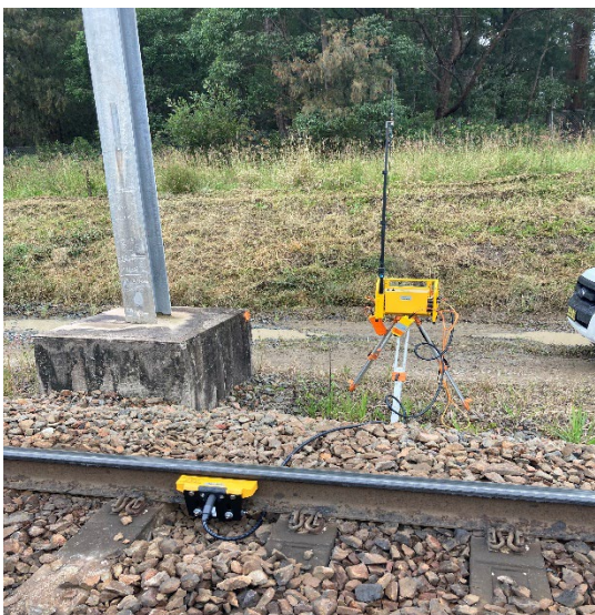
Image 1: Transmitter and sensor installation location
