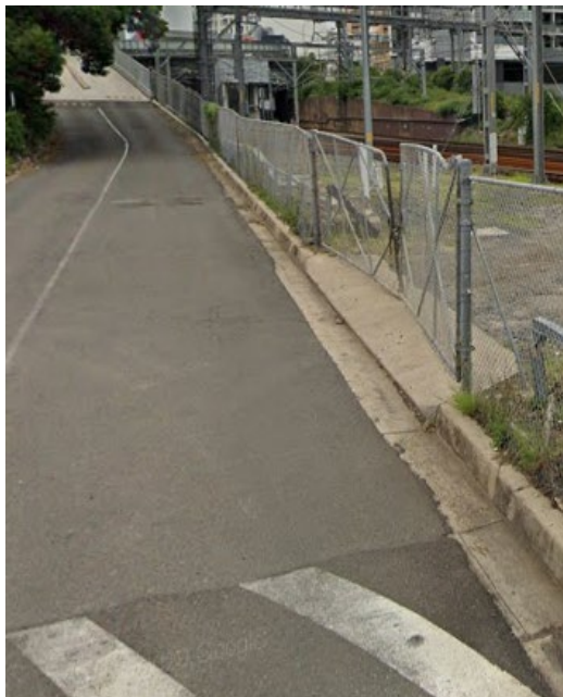
Image 5: Access gate (100 15.037 U) opposite Hurstville Substation
