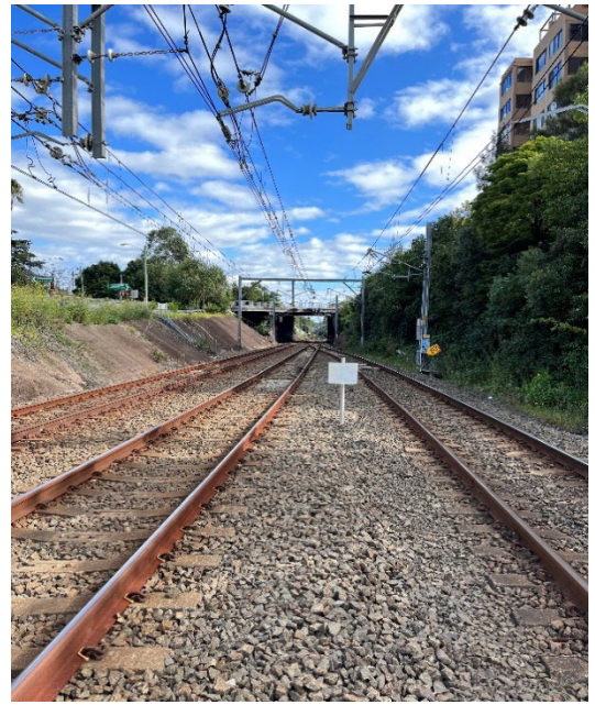
Image 4: View towards 1 & 2 Platforms Penshurst
