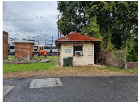
Image 4: Emergency Assembly Point at Clyde Signal Box.
