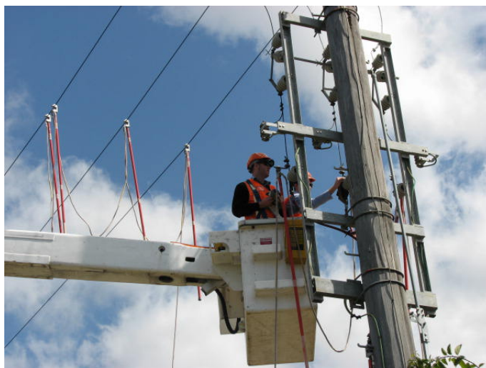
Figure 2 – Example of Installed Aerial Line Earthing Set
