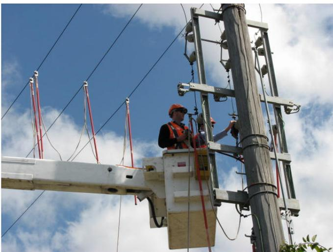
**Figure 2 - Example of Installed Aerial Line Earthing Set**
