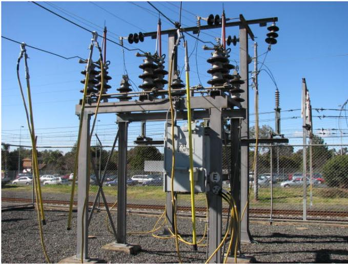
**Figure 1 - Example of Installed Substation Earthing Set**
