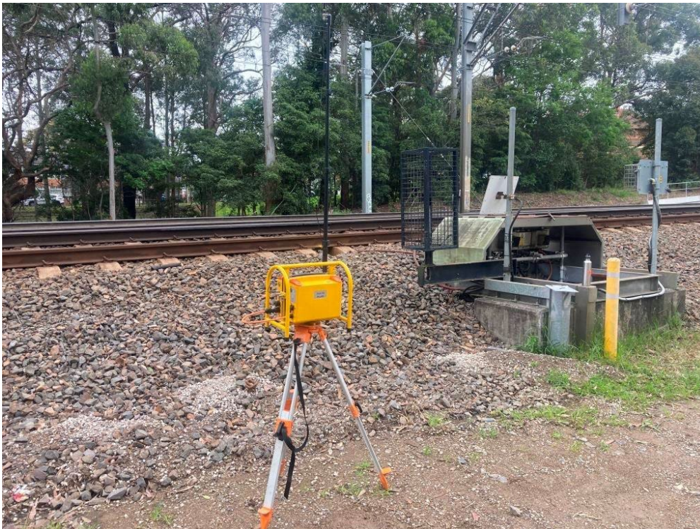
Image 1: Worksite location and ATWS warning unit setup location.
