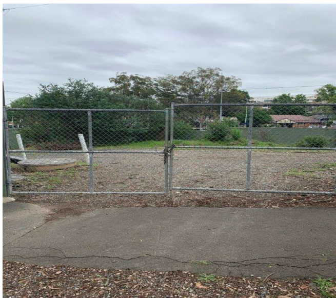
Image 1: Access gate N00 27.084 U.
