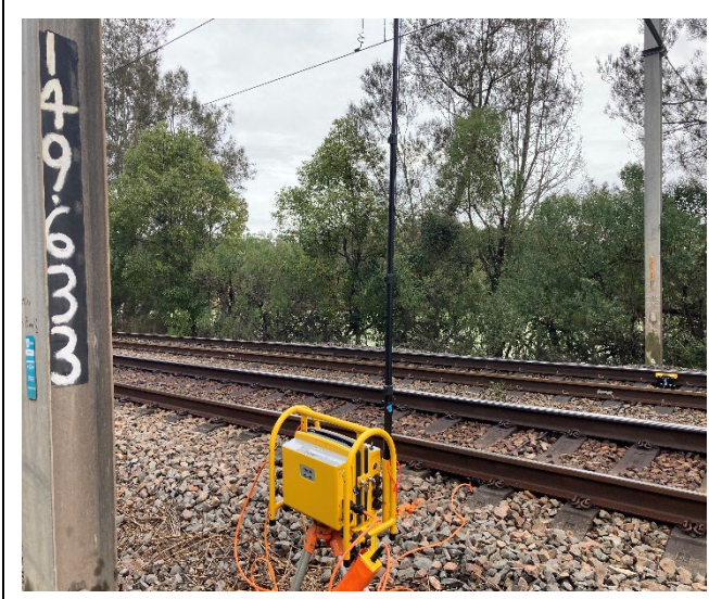
Image 1: Transmitter and sensor installation location
