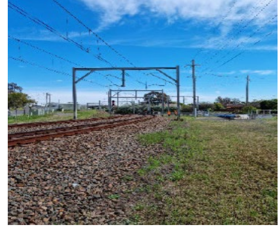
Image 4: View of 22.666 KM location from 22.583 KM.
