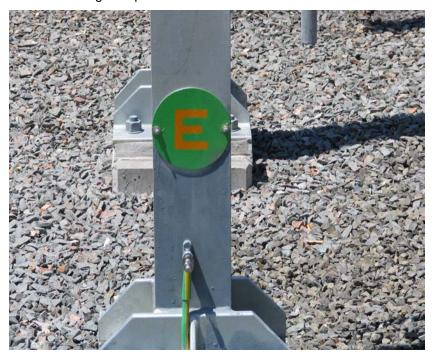
Figure 11: Typical Substation Earthing disc and Earthing Point
