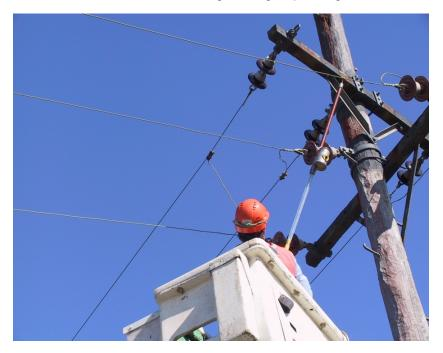
Figure 2: Testing with High Voltage detector
