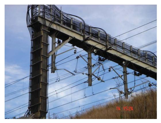
Figure 3: An example of a feeding arrangement from the Substation to the Overhead Wiring
