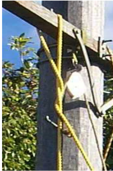
Figure 5: Rescue rope over cross arm with tail one turn around fall of rope
