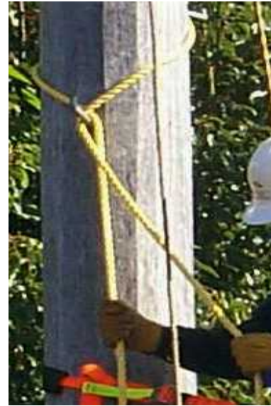
Figure 6: Rescue rope over pole step, around pole with the tail looped over first pole step
