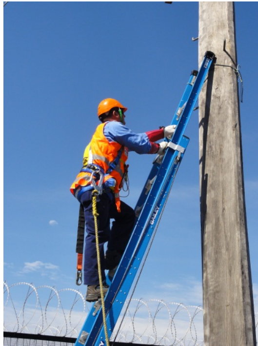
Figure 4: Accompanying Person ascending pole for rescue
