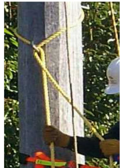
Figure 2 – securing a rescue rope
