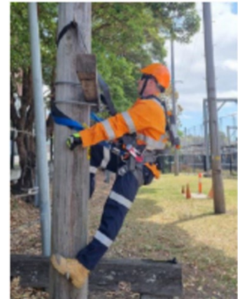
Figure 1 – Attached Climbing with two pole straps
