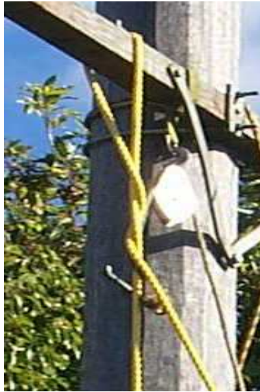
Figure 5: Rescue rope over cross arm with tail one turn around fall of rope
