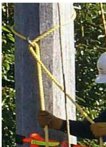
**Figure 2 – Rescue rope using pole peg**
