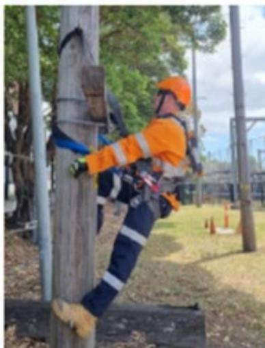
**Figure 1 – Attached climbing with two pole straps**
