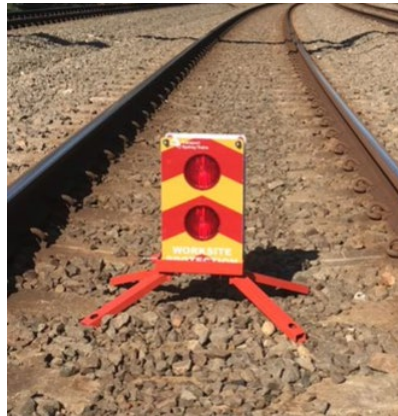
FIGURE 1: A Worksite Protection Marker placed 500m from a worksite inside an LPA
