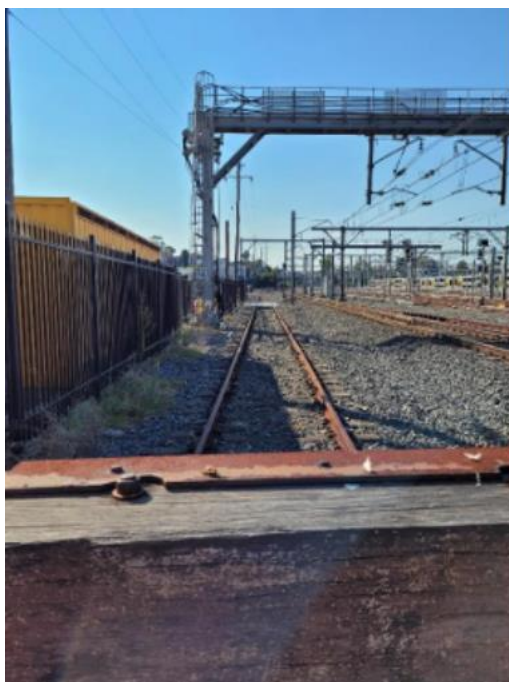
Image 3: View of Buffer Stop at City End of Terminal Line for No.2 Down siding.
