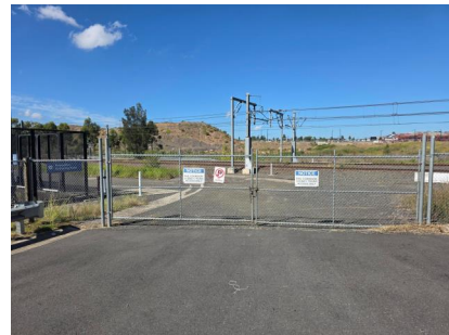
Image 3: Inner HS Access/egress Via Gula Court (Edmondson Park) M28 45.267 to protection placed at 45.055 KM
