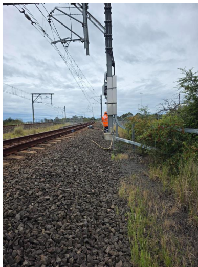
Image 4: Outer HS Location to protection placed at 42.555KM
