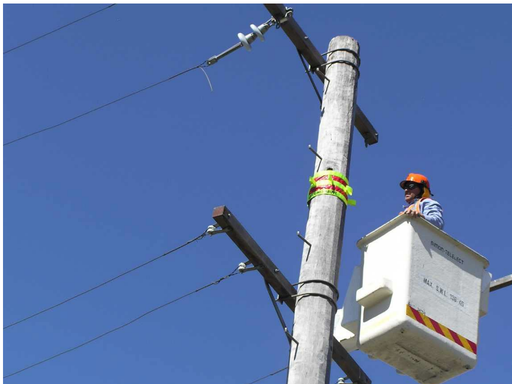
Figure 3: Applying the pole marker from EWP
