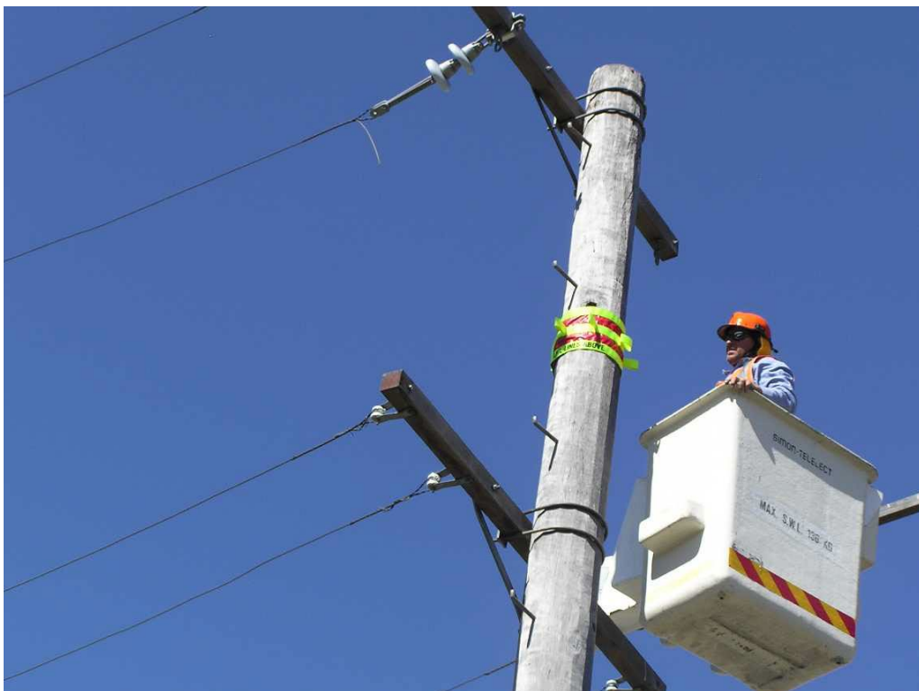
Figure 3: Applying the pole marker from EWP
